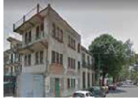
Calle Heroes Vacant building next to Casa Rivas Mercado
