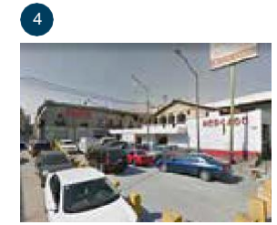
Mercado dos de Abril public space surrounding the market is dominated by parking
